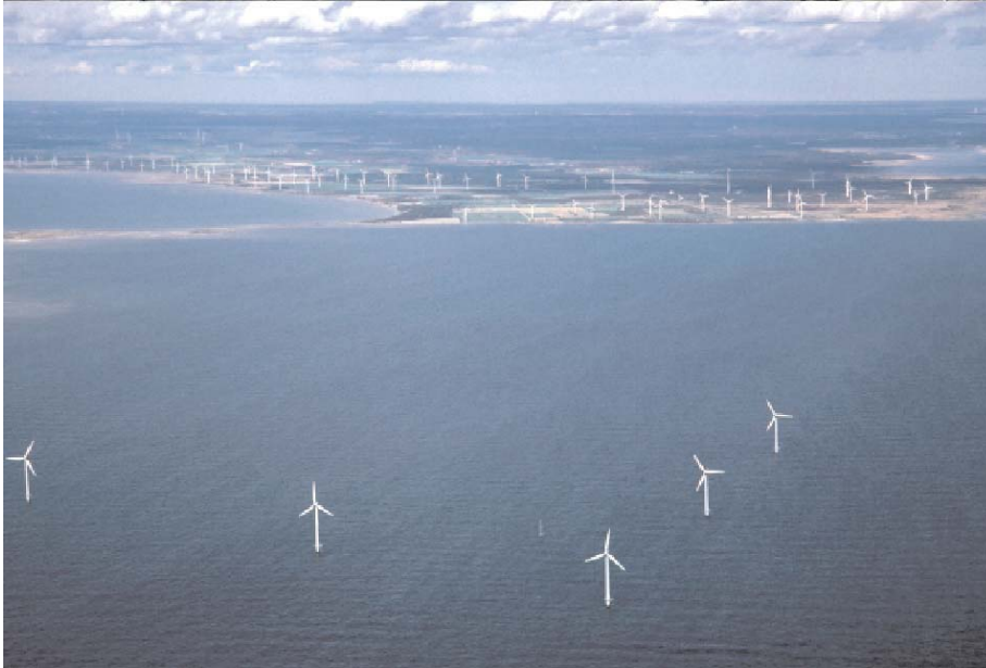
Figure 10. Bockstigen offshore wind farm, Sweden
