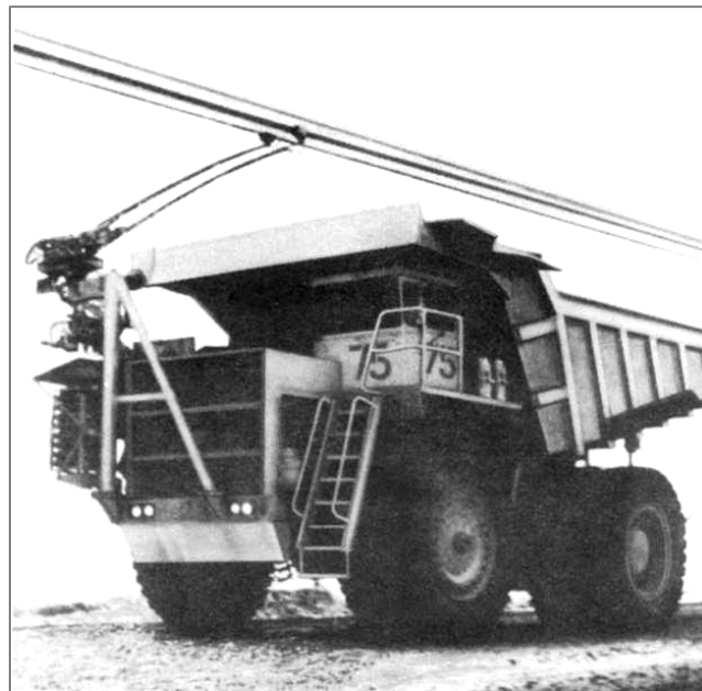
Figure 4. Trolley truck operating at the Quebec Cartier iron ore mine, Lac Jeannine, 1970s.
